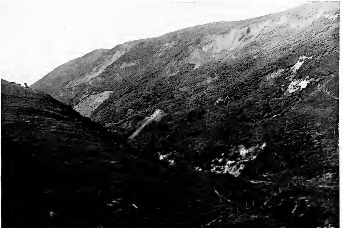
A. Earth-avalanches on side of canyon near Chittenden. A. C. L.
